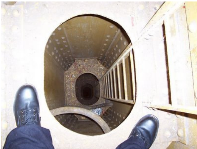
Looking three hundred feet down inside the southwestern tower chamber. The chamber itself is 3' x 4' x 11' high. The opening is 18" x 24"
