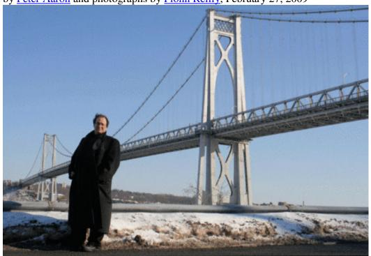
The Franklin D. Roosevelt Mid-Hudson Bridge is a deck-truss, gravity-anchored suspension bridge designed by Polish immigrant Ralph Modjeski and completed in 1930 at a cost of \$5,900,000. A formidable 3,000 feet long and 39 feet wide, it rises 135 feet above the Hudson River. Connecting the hamlet of Highland to the city of Poughkeepsie, it stands as a true marvel of modern engineering. It's a vital commuter conduit, an instantly recognizable local landmark, and a...musical instrument?
